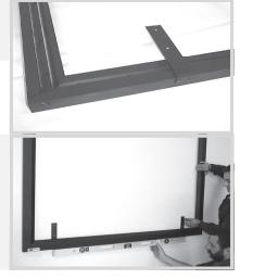
STEP 4. It is recommended that you utilise three brackets each on the top and bottom of the frame, although side fixing in conjunction with bottom brackets would also be acceptable practice.
