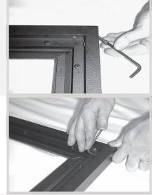
STEP 6. You will see connected to the bottom corner of the side frames an angle bracket that now requires bolting to the bottom frame using the M5 nut and bolts provided. The lower half of your frame in now complete, now to assemble the top section.
