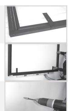
STEP 7. With all four brackets attached, place screen frame (not with surface) on the wall and mark holes.
