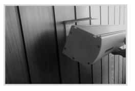
STEP 7. Ensure projection screen case is latched into the bracket as shown.
