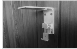
NB: Top of bracket equals top of screen canister.
