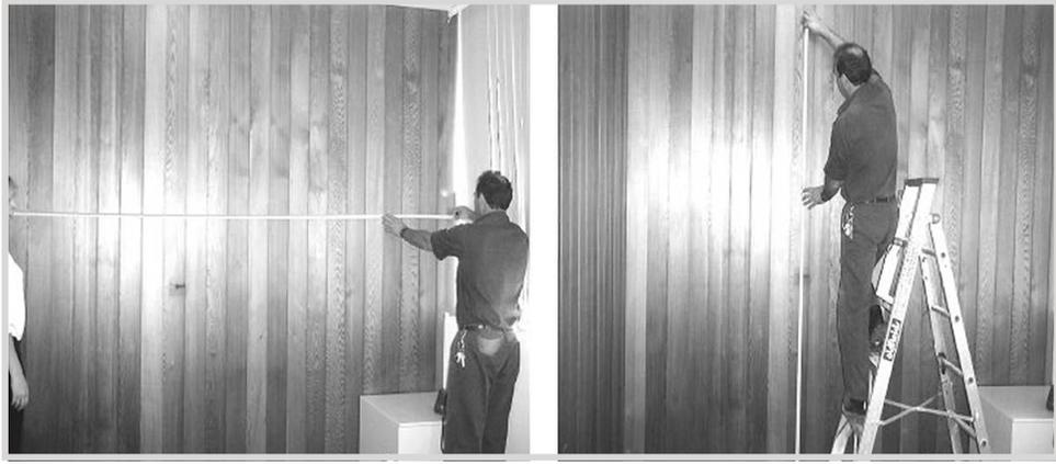
**STEP 2.** Measure the length of screen canister along the top surface and mark the centre of the canister with a pencil, to assist in lining up the screen when mounting.
