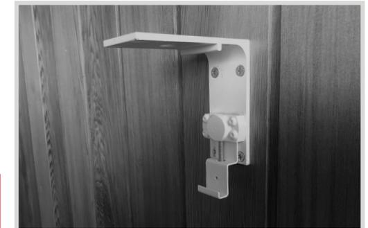
NB: Top of bracket equals top of screen canister.
