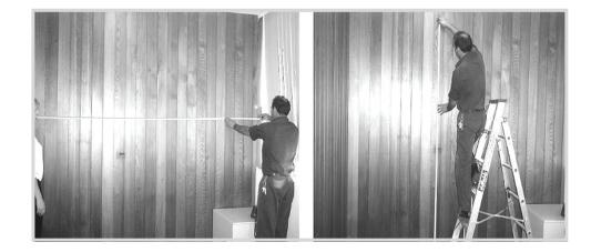
STEP 2. Measure the length of screen canister along the top surface and mark the centre of the canister with a pencil, to assist in lining up the screen when mounting.
