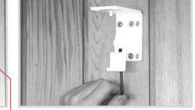
NB: Top of bracket equals top of screen canister.
