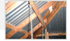
STEP 2. A minimum of 4 points to secure the chain is required and it is the installers responsibility to ensure the chain turnbuckle system chosen is strong enough for the safe installation of the unit.
