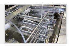
STEP 2. Lay out the required cables and lock them into position utilising cable ties in the small regular holes running up the channel.
