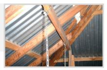
STEP 3. Secure the chain to a suitable structure, such as overhead timber beams, or dyna-bolted to an overhead concrete slab.
