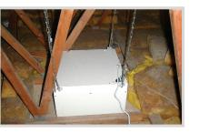
STEP 6. Raise the unit into the ceiling, fit the screws or bolts (as appropriate to selected method) and apply upward pressure to the unit so the ceiling edge trims are pressed firmly against the underside of the ceiling material and tighten off the screws or bolts.
