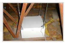
STEP 3. Wind a set of nuts up the rods above the installation height and then insert the rods through the supplied angle brackets, now attached to the lifter unit.
