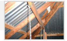
STEP 2. A minimum of 4 points to secure the chain is required and it is the installers responsibility to ensure the chain turnbuckle system chosen is strong enough for the safe installation of the unit.
