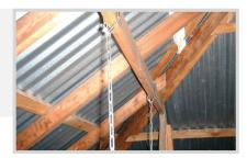
STEP 2. A minimum of 4 points to secure the chain is required and it is the installers responsibility to ensure the chain turnbuckle system chosen is strong enough for the safe installation of the unit.
